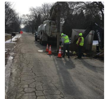
Sewer Main Repair
